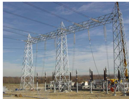
Figure 5: Overhead line cables transition station (400kV)
