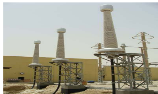
Figure 6: 400 kV Termination under construction
