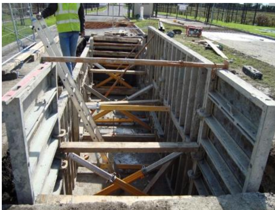
Figure 2-9: Typical joint bay under construction (in-situ)
