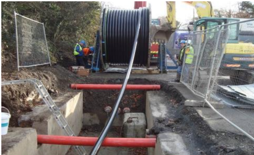
Figure 2-12: HV cable pulling procedure (Typical drum set-up)
